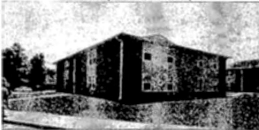
Skiatook (Prior to Rehabilitation)
