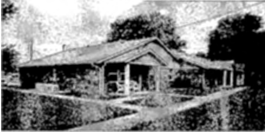
Wagoner (Prior to Rehabilitation)
